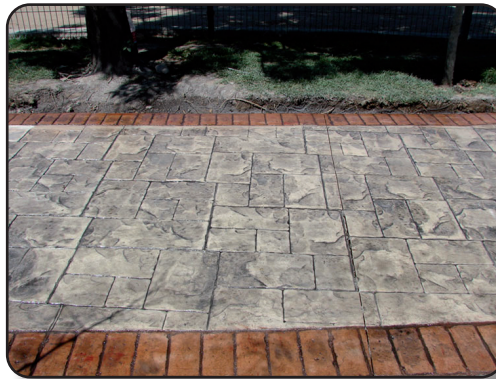
Acid for decorative concrete
